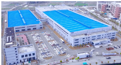
● Exterior of the intelligent factory.
